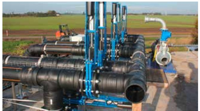
**At Gemidan's pre-treatment plants, food waste is converted into a pure bio pulp. Their technology ensures a sustainable use of the waste, and AVK knife gate valves control the flow.**
